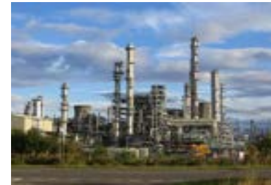
Petro Chemical G Plant Project & Goods Clearance
