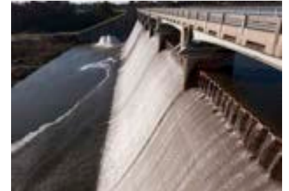
Dam Construction Projects
